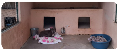
The kennels BEFORE the work
