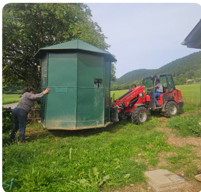
Removal of the former aviary
